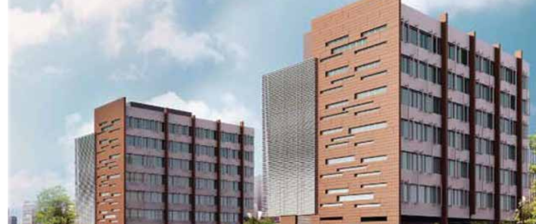
Martin Burn i-space (I - II), IT/ITES Building at New Town behind Tata Memorial Hospital, Kolkata.
